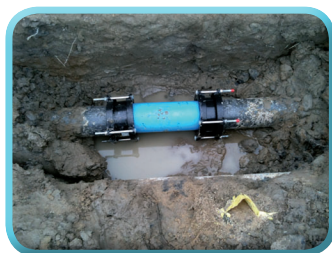
Repaired Leak
